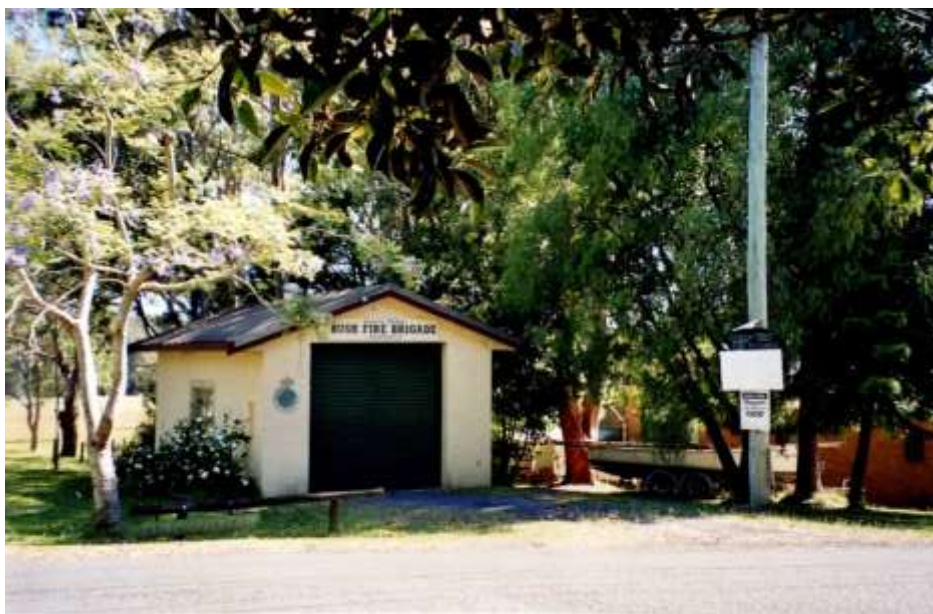
Old Fire Brigade Hall
